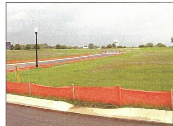
Temporary seeding involves the establishment of rapid-growth annual grasses or small grains to stabilize disturbed areas until such time as a permanent, non-erosive cover can be established. Mulching is the application of plant residues like straw or wood chips to enhance and protect vegetative establishment and minimize erosion potential.
