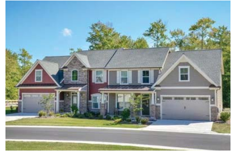
Two attached single-family homes.
