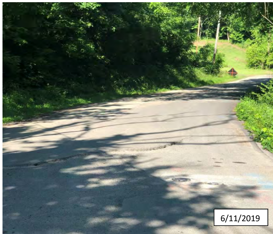
Photograph #2: Looking west along Dillsboro Road near east end of project.
