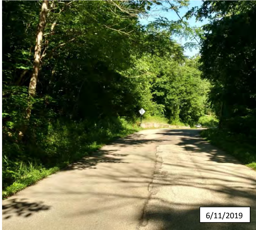
Photograph #5: Looking west along Lower Dillsboro Road near west end of project.
