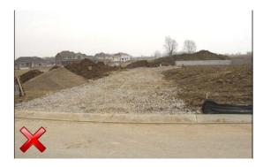
Example construction entrance at a small site. Notice the accumulation of sediment in the rock has resulting in transport onto the roadway. No diversion berm was installed to prevent sediment-laden runoff from flowing onto the roadway. Also note that the silt fence has not been properly turned uphill to prevent sediment washing onto the entrance and/or onto the public roadway.
