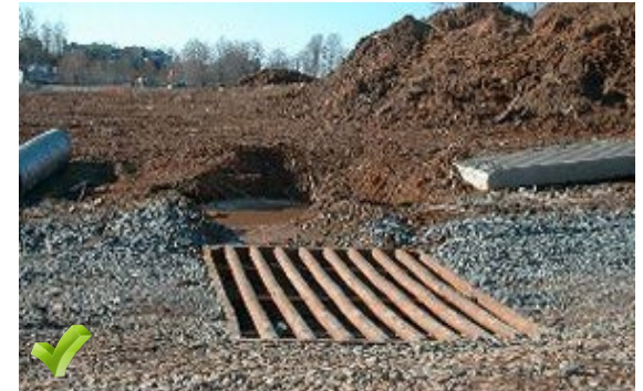
Example of a wet pit used for hosing of vehicles to minimize sediment deposits on the roadway. Note: The sediment collection traps must be periodically cleaned to remove accumulated sediment. Tire runoff must be diverted to an area on the site where it is detailed. These traps are only intended to collect sediment; they are not for excessively oily or greasy equipment.
