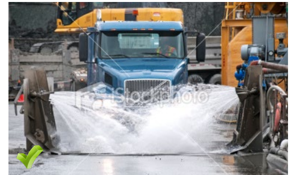
Larger sites that are hauling significant amounts of material to/from the site are better managed through more significant vehicle washing measures.
