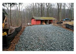
Construction entrances are access points to the site that are designed to dislodge sediment from tires before construction vehicles enter the roadway.
