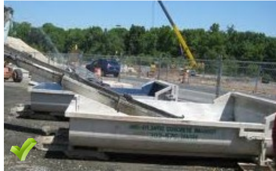
Self-contained sturdy containment systems that are delivered to a site and located at strategic locations for concrete washout.
