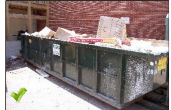
Majority of the construction waste is contained inside the dumpster. Liquids should never be emptied in the dumpster.
