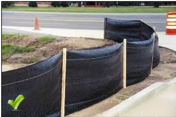
Silt fences should be installed and maintained in disturbed areas to collect sheet flow runoff from the site. Never place a silt fence across concentrated flow, such as a ditch, swale, or drainage channel.
