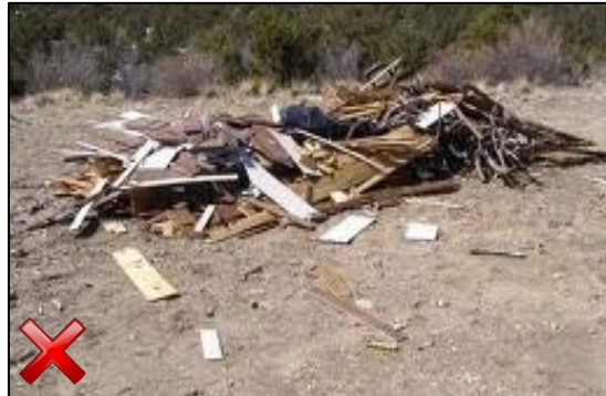
Properly dispose of construction waste into a provided dumpster. Pick up garbage to prevent items leaving the site. Make sure dumpster remains closed at all times to prevent exposure to rainwater.
