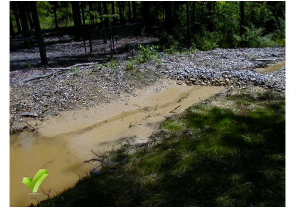
Good application of sediment trap installation. The stone spillway provides a stable overflow structure. Sediment basin is at capacity and should be cleaned prior to next storm event.
