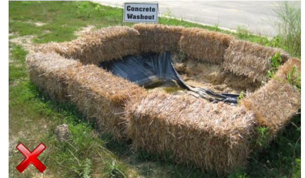
The polyethylene lining should wrap over the straw bales and be properly secured along the top. The lining used at this washout area is not thick enough.
