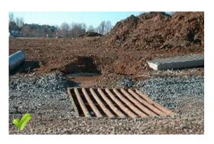
Example of a wet pit used for hosing of vehicles to minimize sediment deposits on the roadway. Note: The sediment collection traps must be periodically cleaned to remove accumulated sediment. Tire runoff must be diverted to an area on the site where it is detailed. These traps are only intended to collect sediment; they are not for excessively oily or greasy equipment.
