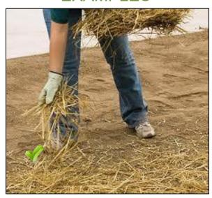
As soon as feasible, sites should be temporarily stabilized with straw, or permanently stabilized with grass and sod. When straw is used, it should be crimped or "punched" into the ground to prevent the straw from moving during wind and rain events. Erosion control mats or sod should be used in concentrated flow areas, such as ditches and swales.
