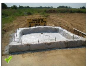
Contractors and subcontractors should utilize concrete washouts whenever pouring or placing concrete or mortar. Washouts should be used for rinsing off mortar and concrete mix, process and placement equipment. It is not acceptable to wash off equipment outside of a contained concrete washout area.
