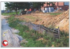
Inadequate maintenance of silt fence.
