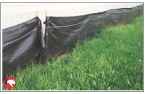
Two sections of silt fence not properly connected. Sections should be overlapped and wrapped together.
