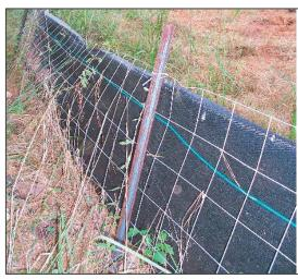
Use wire-reinforced silt fence and steel posts to reinforce sections downstream of large areas.
