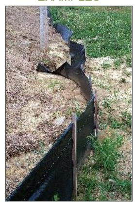
This silt fence is still functioning, but in need of cleaning and replacement.
