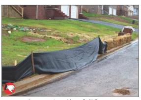
Improper trenching of silt fence.
