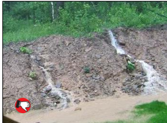
Temporary seed and mulch not applied to the slope. Erosion of soil occurs during rain event.
