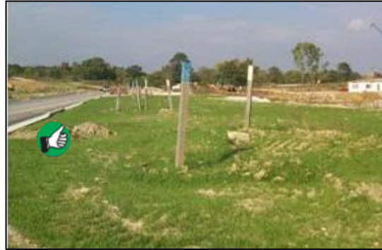
Example of temporary seeding to cover open areas where construction is not taking place.
