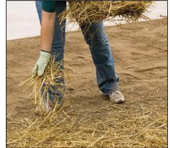
Straw mulch being placed by hand over bare soil.
